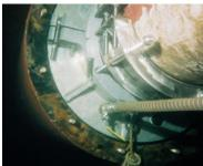
Above: Diver working inside inflatable habitat (top). The inflatable habitat is fitted around the stern seal area creating a water tight fit (second).
